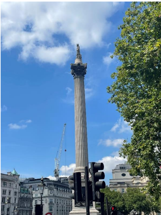
Nelsons Column (about to topple) Trafalgar Square
