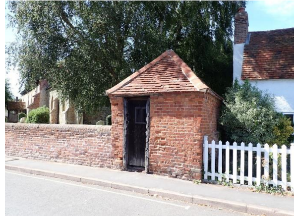
Local Jail - Bradwell
